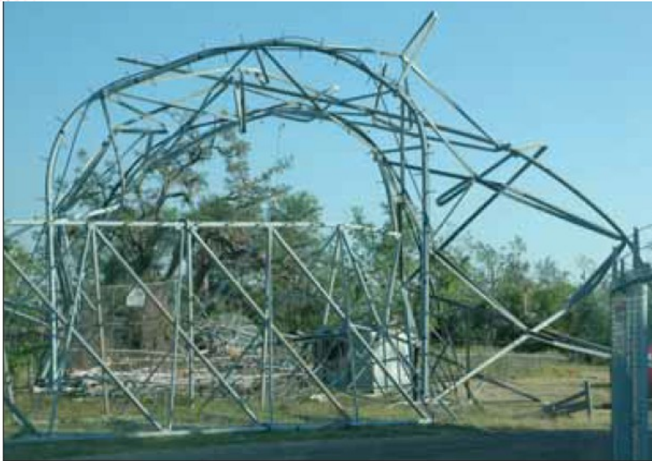
A downed communications tower, Plaquemines Parish, LA.
