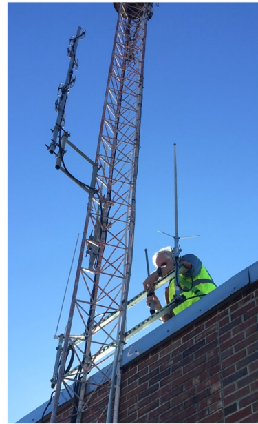
Art Grant installing new microwave MESH antenna/transceiver.
