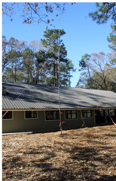
Net Control—Bear Lake Campground Pavilion WB6IQN Dual Band J-POLE @ 35 FEET
